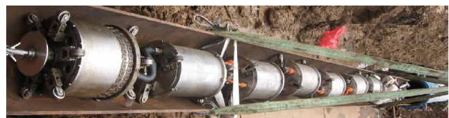
Figure 12 The in-pipe robot being introduced into the pipeline for field tests
